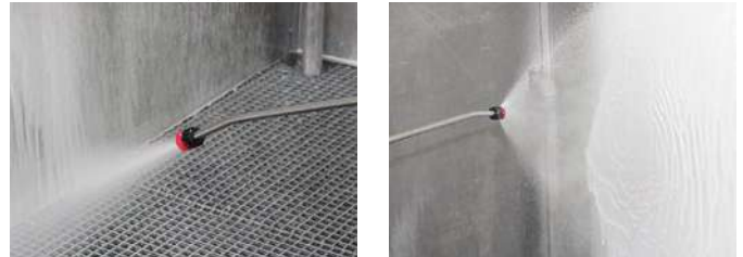
Applying cleaner with compressed-air foam lance
